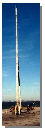
A.D.S. has experience in designing equipment and installing wick drain to depths of up to 260 ft. A.D.S. has also installed wick drain in all types of soil conditions.
